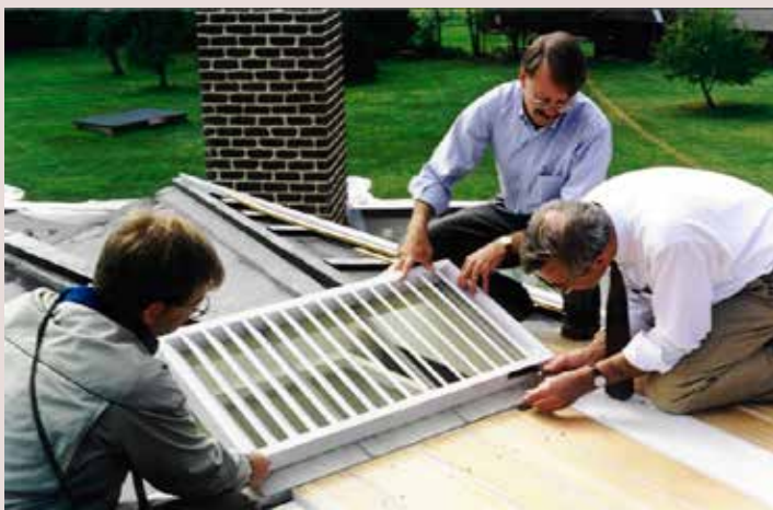
Fitting skylight blinds: L-R: Jeff Baker, Travis McDonald, John Mesick, 1997
