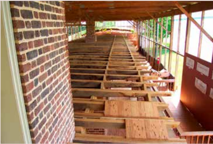
Above: Oak joists for Jefferson's special terras roof of the east service wing, 2005
