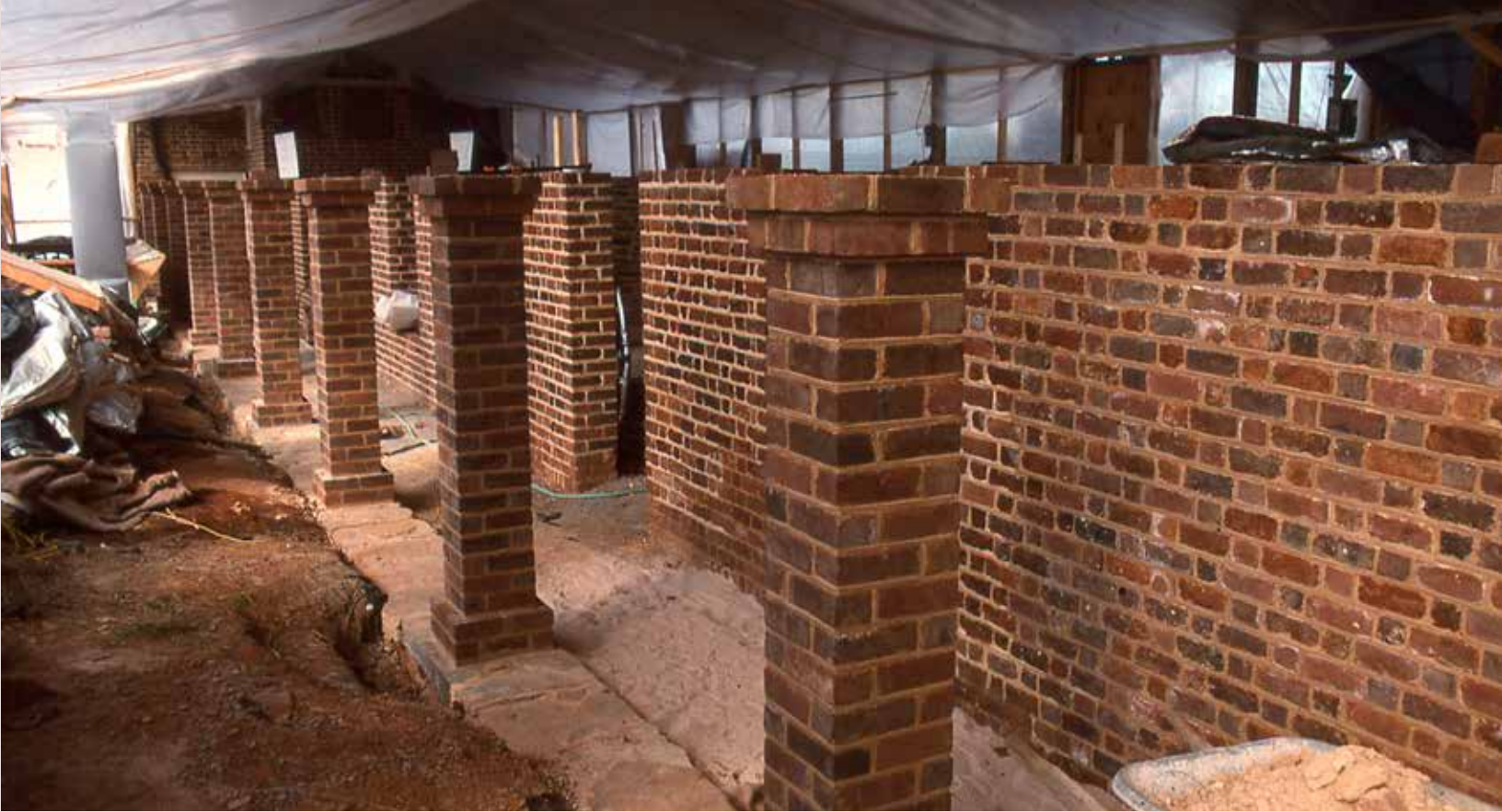
Walls of the east service wing reconstructed and restored, 2004
