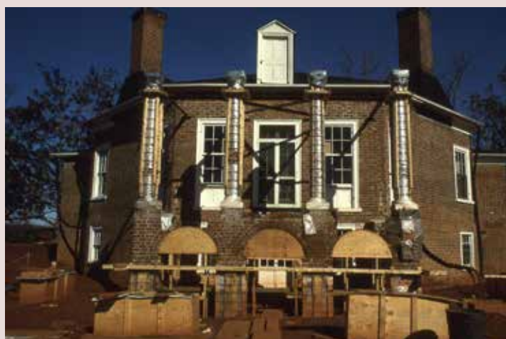
South portico during repairs to arches and columns, 1993
