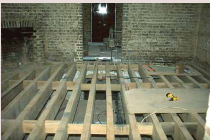
New oak floor joists installed in the center dining room, 1999
