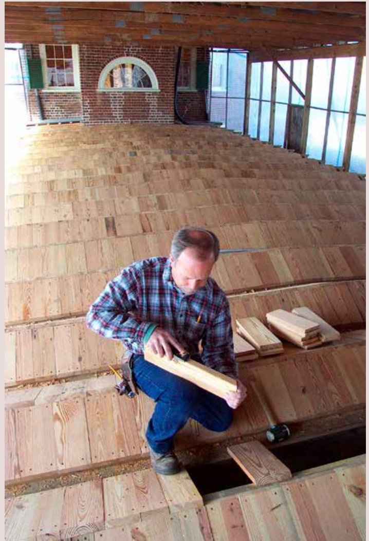
Left: Vince Fastabend uses an adze on the east service wing joists. 2006
