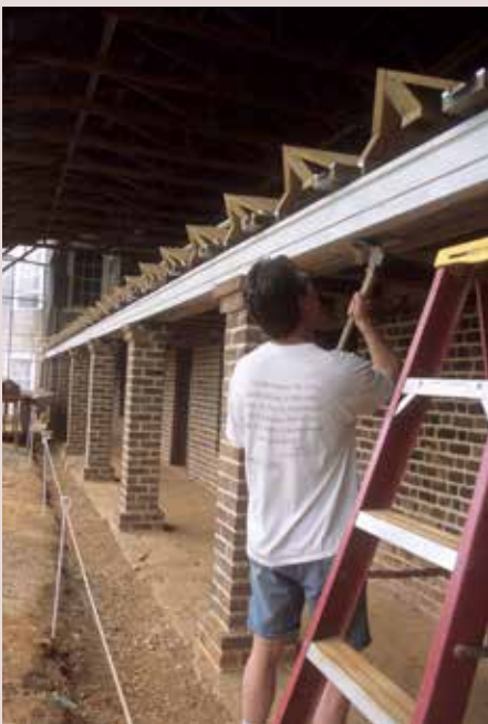
Above: Oak joists for Jefferson's special terras roof of the east service wing, 2005
