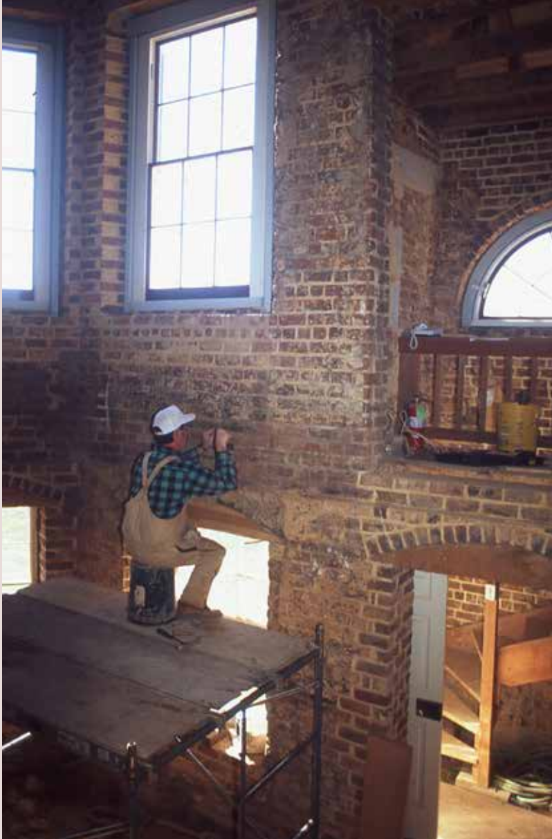
Wayne Mays repairs brick joist ledge, 1997.
