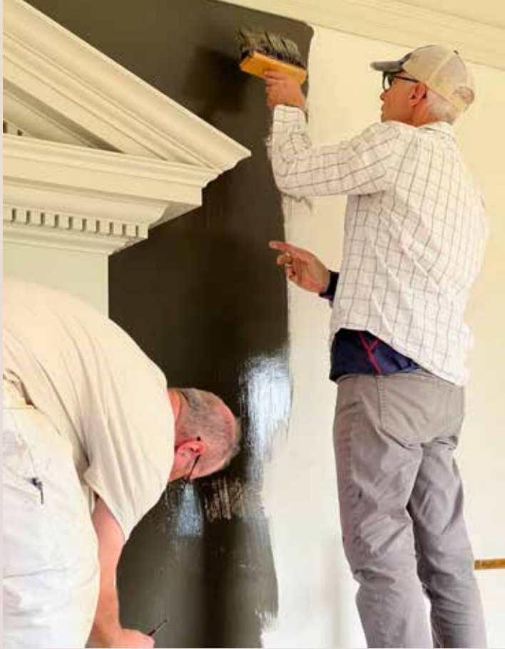
Handmade distemper paint goes on the parlor walls, 2022
