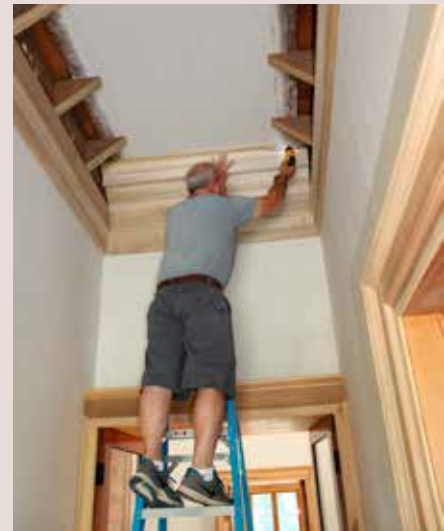
Dave Clauss installs the large Tuscan Order entablature molding in the passage, 2016.
