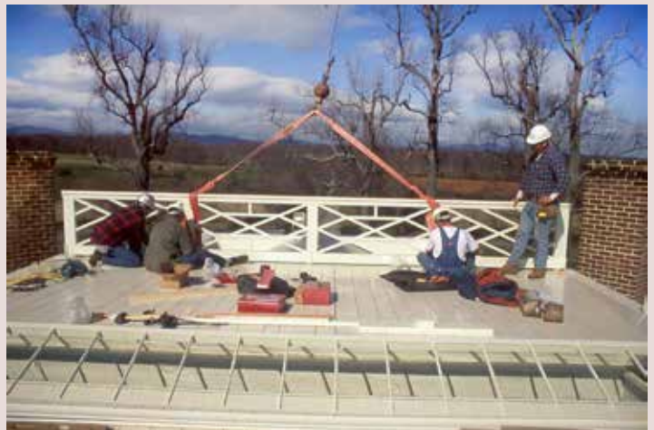
Installation of Chinese Railing on upper terras roof deck, 1998
